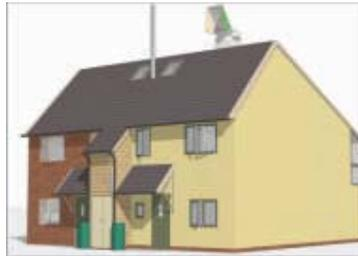
photovoltaic panels (PV) have been included on the roof to accommodate the electrical demand from lighting, pumps and fans and all the domestic appliance load.
